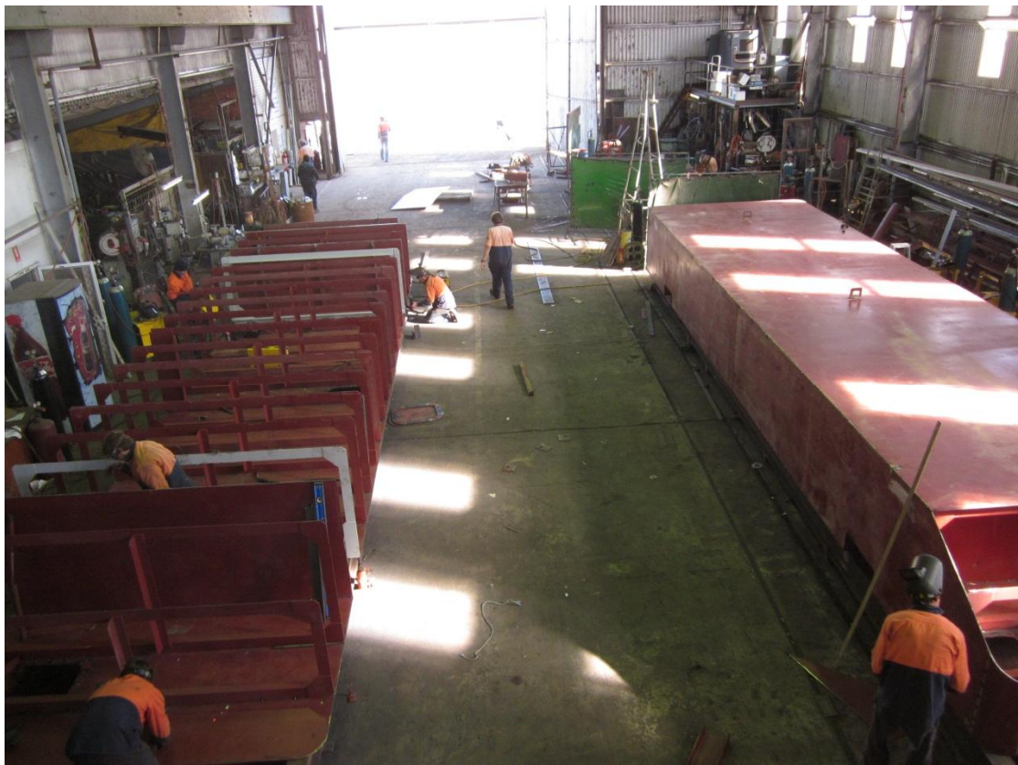
Photo 16 Existing slipway indoor construction areas
