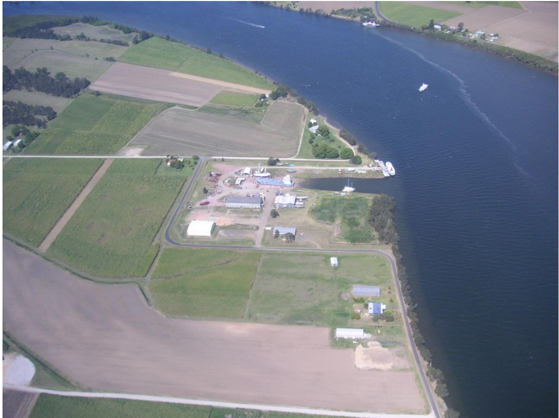
Photo 19 Existing slipway with proposed marine precinct in background
