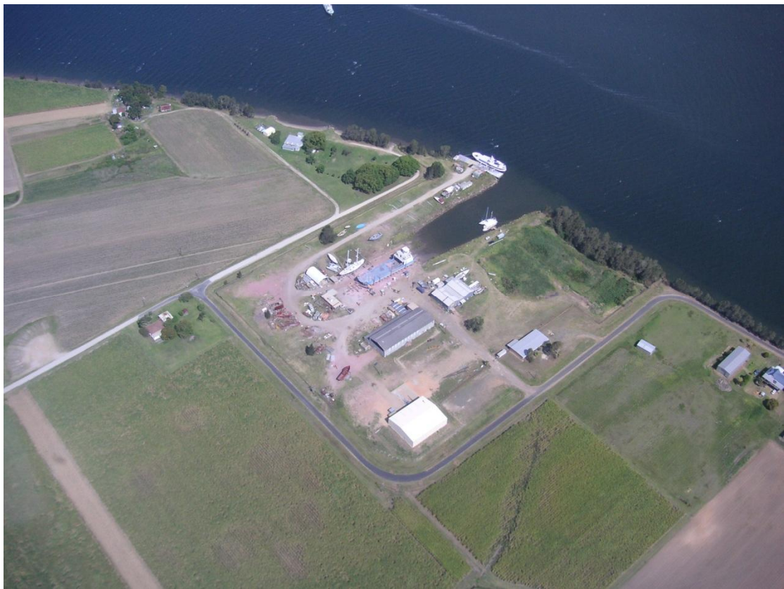
Photo 18 Existing slipway in 2008
